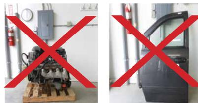
In your facility, there must be a minimum of 36" (3 feet) of clearance around electrical panels serving between 120 and 250 volts. Circuit breakers must be clearly labeled with accurate and current directories.
